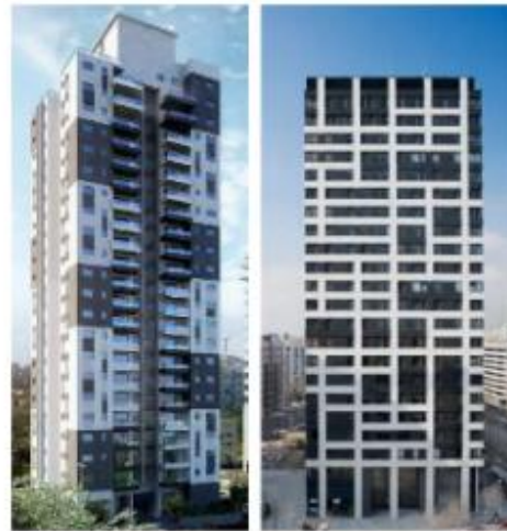
nova diagonal tower, Barcelona, MSA+AC MSA+AC GROUP
